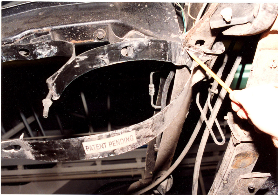
30. Close-up view of the rear tank strap for the failed CNG highlighting a tear in the strap adjacent to the bottom flange of the left frame rail
